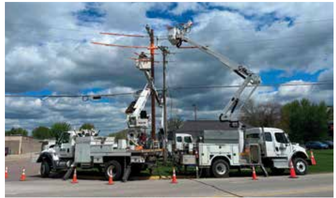
Vernon Electric crews establish a roadside work zone while completing line work. Drivers should slow down, move over when possible, and remain alert when approaching utility vehicles.
