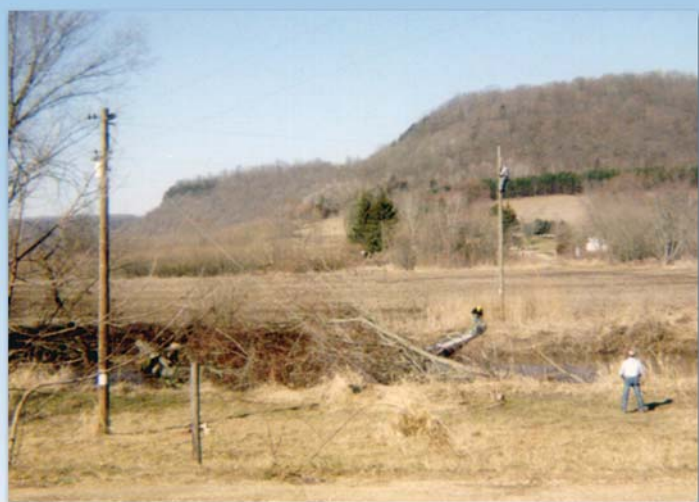
Trading a Work Truck for a Work Canoe —High waters on the Kickapoo River this spring caused a large tree to fall along the bank between Viola and Readstown near Kickapoo Corners. The tree came down on a Vernon Electric distribution power line crossing the river and serving the area, causing a widespread outage. The fallen tree pinned the fallen wire in the Kickapoo River. Since the far side of the river was not accessible by vehicle, linemen had to leave their truck behind in favor of a canoe to clear the tree and cross the river. Pictured in the canoe are Mike Burger and Charlie Burch.
